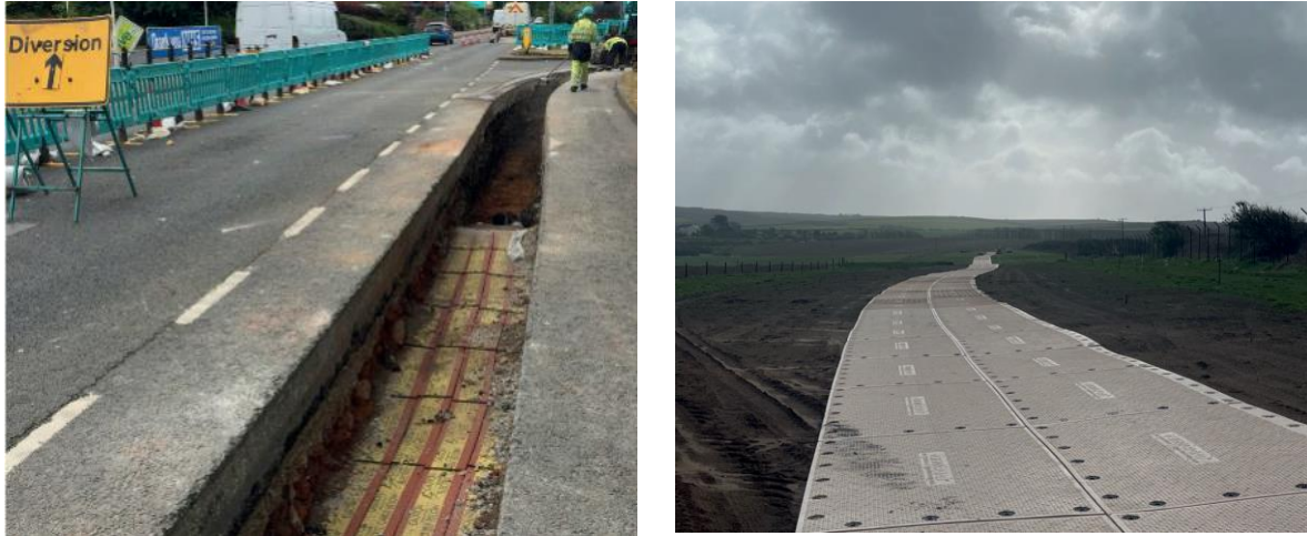
Figure 4.4: Cable installation in Wales
